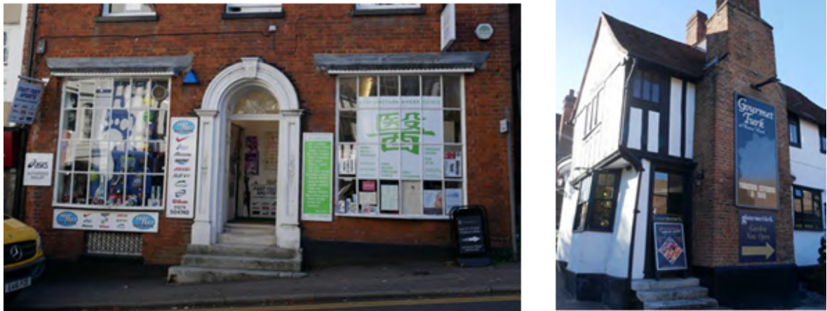
Figure 38 – Excessive signage significant in number and scale.
