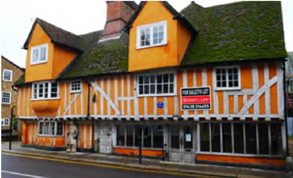
Figure 13 – The 15th century jettied, timber-framed building, St. Nicholas Hall or Verger's House accommodating retail.
