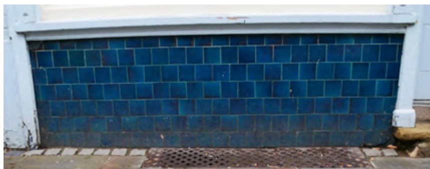
Figure 30 - Glazed blue tiles appropriate to this stallriser.
